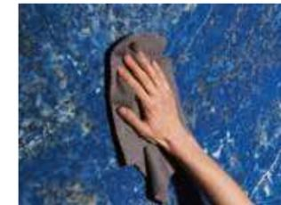
White body ceramic tiles can be cleaned with a simple passage of hot water or neutral detergent.
